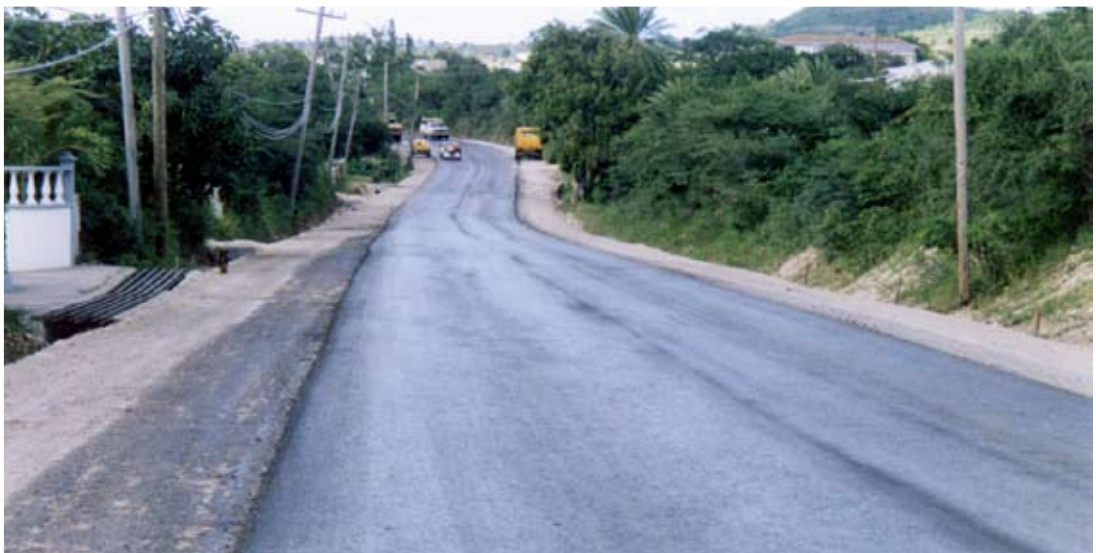
Reconstruction of all Saints Road Project
