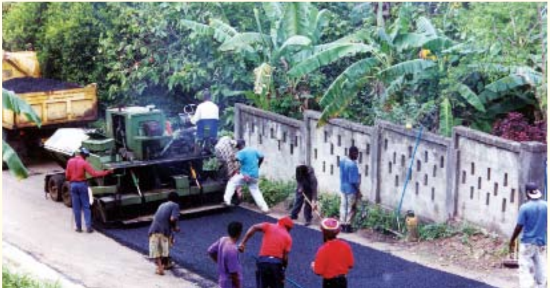
Coastal Defences and Roads Rehabilitation Project
