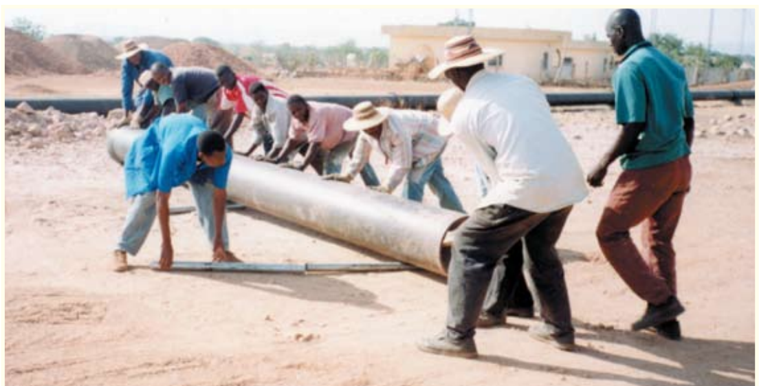
Santiago De Cuba Water Supply System Rehabilitation Project
