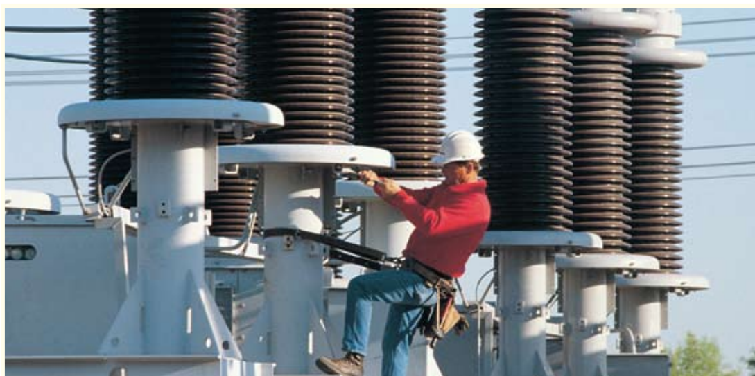
Expansion of Cane Hall Power Plant Project
