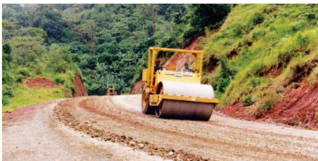
Rehabilitation of Feeder Roads
